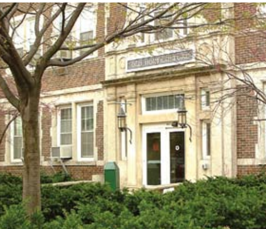
Old Horticulture Hall is one of the buildings used in MSU's classroom rescheduling program to reduce energy consumption.
